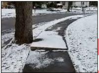
Sidewalk in disrepair creates low spot, trapping water – creating potential icy spot in winter and tripping hazard.
